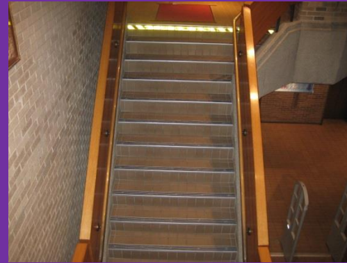
Non-slip stair treads installed, Malpass Library east and west entrances
