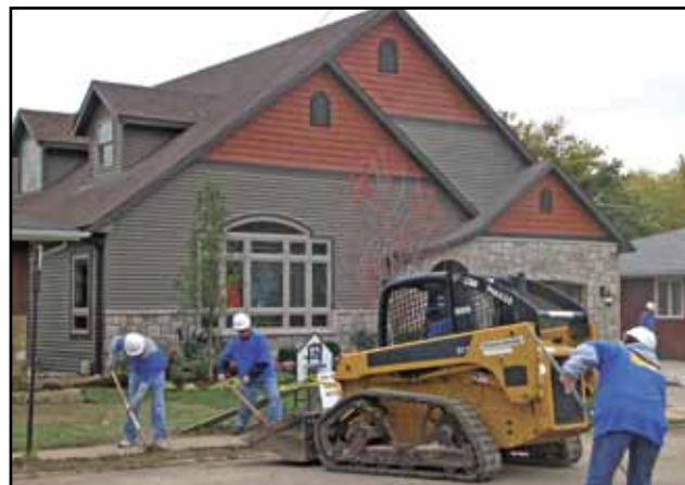
Volunteers helped construct the new home that improves daily life for 8-year-old Jake Grys.
